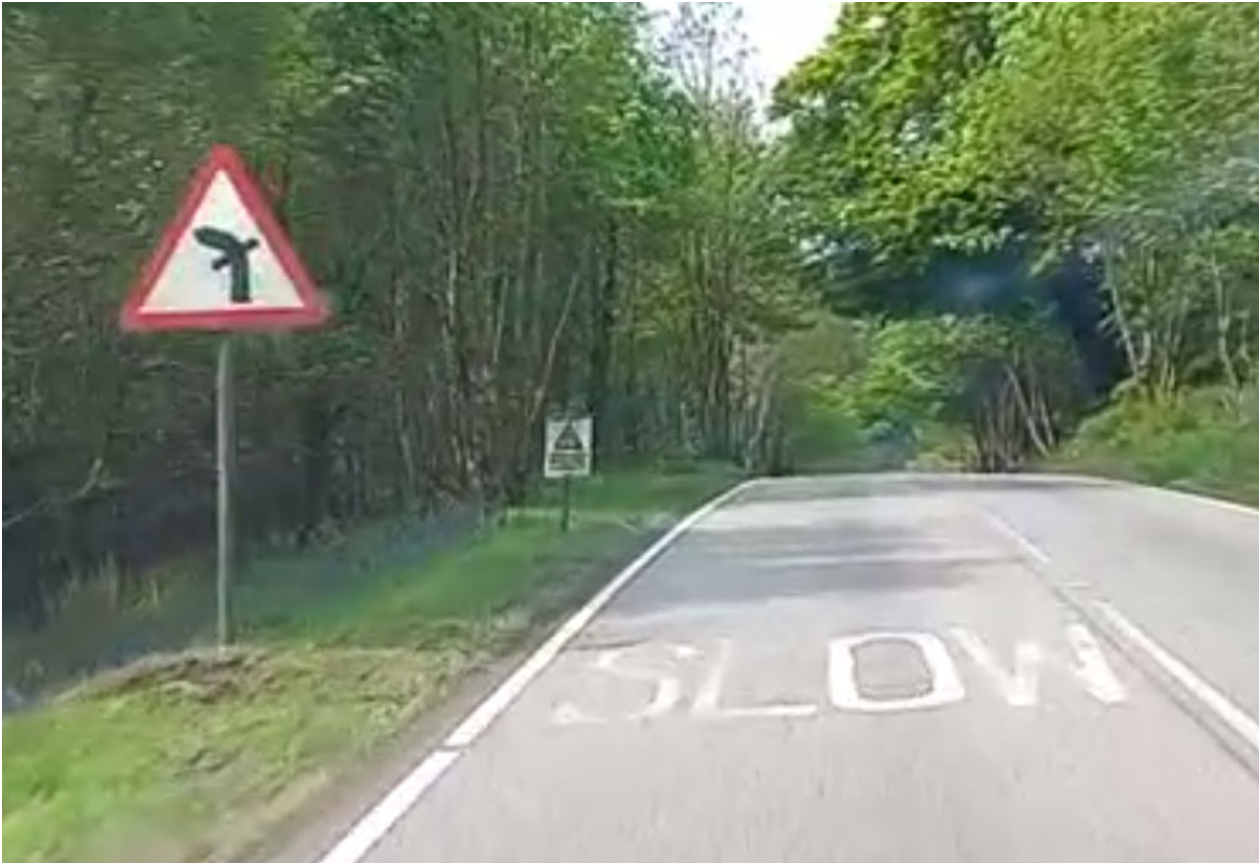
Photo 1: A83(T) east of the existing access - from video footage taken on 22 nd May 2023 – see here: A83 - Google Maps
